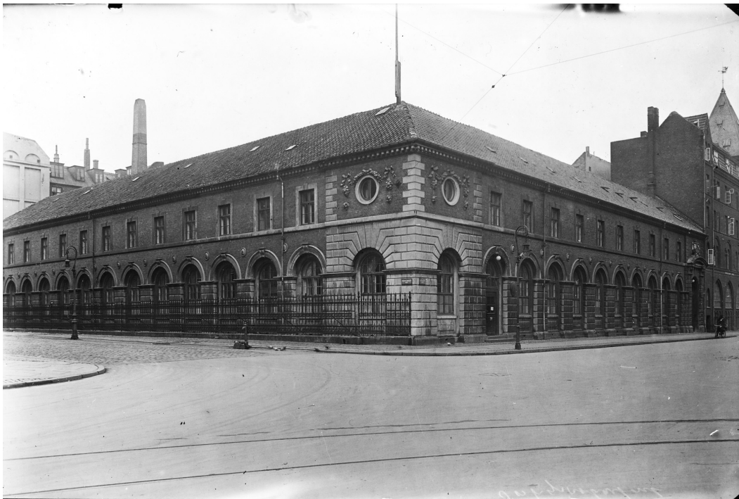
5) The Royal Mint at the corner of the streets Holbergsgade and Herluf Trolles Gade in the centre of Copenhagen. C. 1907-1924. The Mint was built 1872-73 and used for coining 1873-1923. The building still exists, now heightened and used by the SFI – The Danish National Centre for Social Research.
